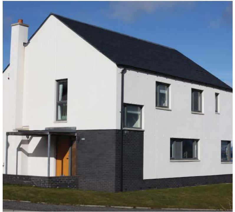
The Drum: A simple palette of white render and engineering brick unifies the development. Canopies, eaves and other projections are minimal and present relatively 'flat' modelling of elevations.
