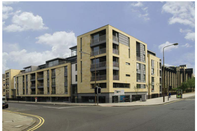
Eyre Place: Eternit cladding panels at ground floor, top floor and accent areas.
