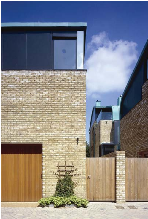
Accordia: street elevations carefully considered to provide vertical articulation.
