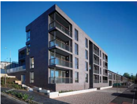
The Botany: Characterful, but simple brick use for flatted accommodation and terraced housing. Sensitive use of flat and pitched roofs. Coherent streetscape and clean street elevation.
